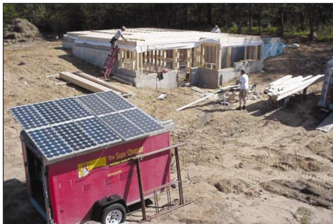
A recent home constructed near Marshfield is a passive solar design with in-floor radiant heat. Below, the "Sun Chaser" trailer set up at a job site provides the necessary electricity for home framing prior to having access to conventional electric hookups.
