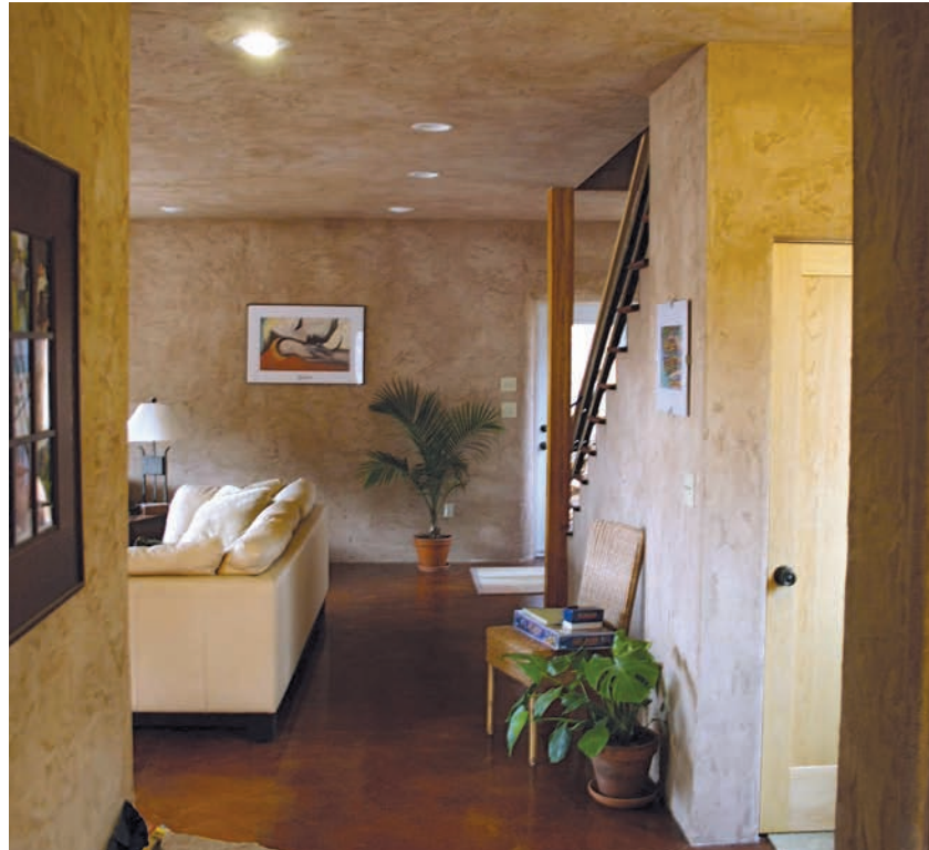
Left: The hydronically heated first floor, before and after the thin-slab concrete was poured. Right: The finished floor and the earth-clay plastered walls help create an elegant, but earthy, atmosphere.
