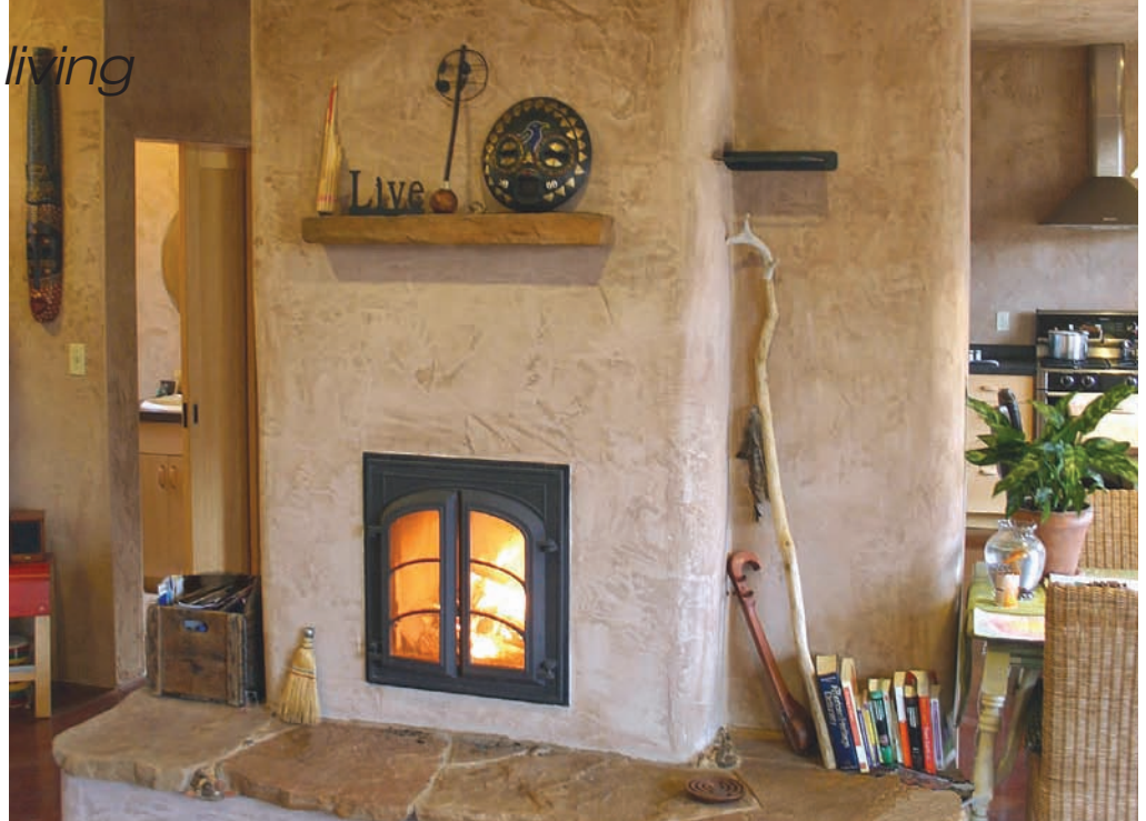
Left: Laying the masonry heater's refractory brick. Right: The final product in action!
